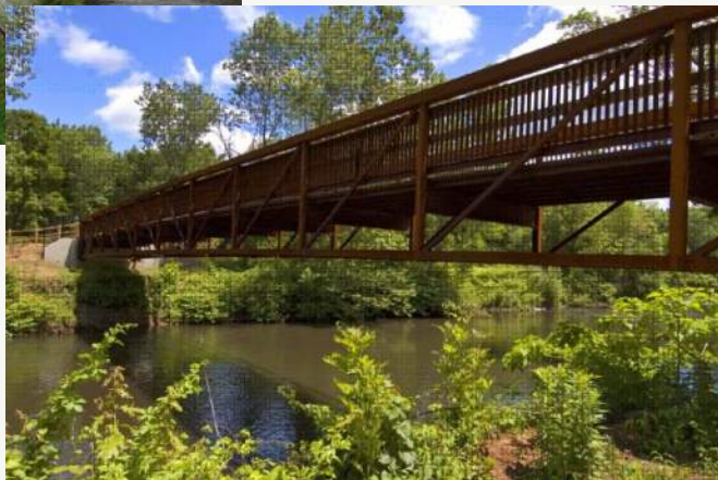
Existing QRLT Pedestrian Bridge Over Quinnipiac River
