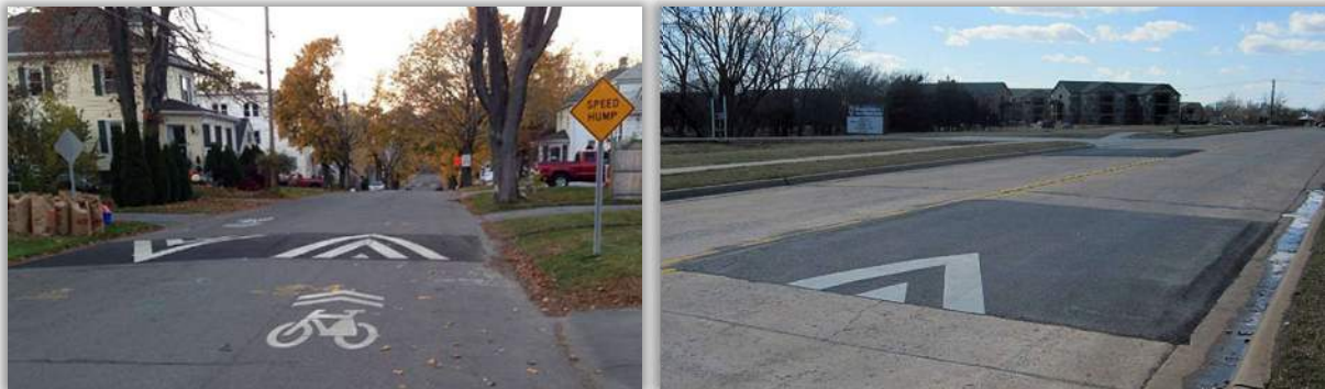
A speed hump and speed table. Source: FHWA
