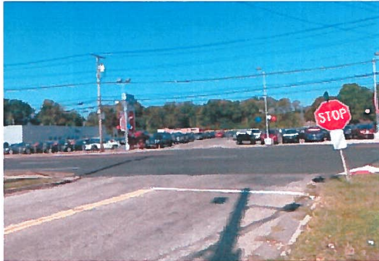
Figure 46: US-1 (Bridgeport Avenue) at Avery Avenue
