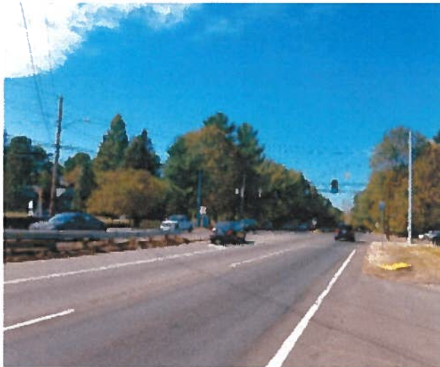
Figure 71: Intersection of CT-34 and CT-152/Orange Center Road (West Leg of Intersection)
