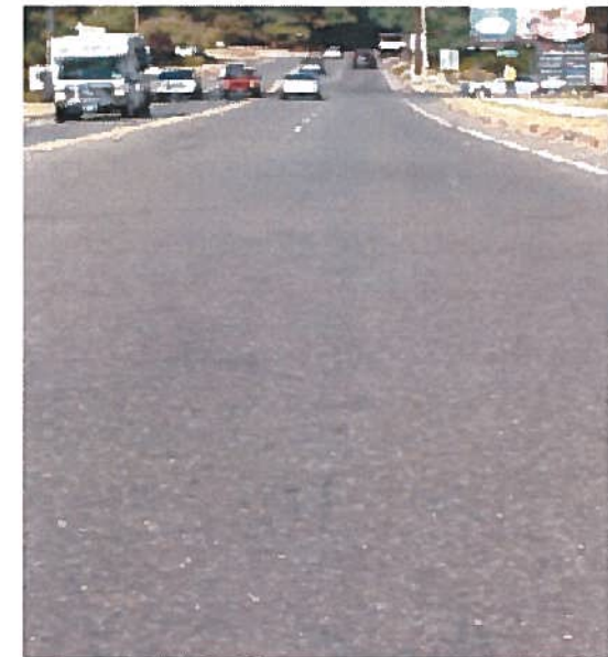
Figure 90: CT-63 approaching Bradley Road
