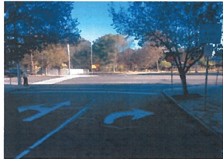
Figure 53: Intersection of State Street and Trumbull Street (Trumbull Street Approach - Facing Interstate On-Ramp)
