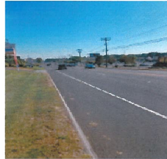
Figure 72: Corridor 30: US-1 (Boston Post Road)
