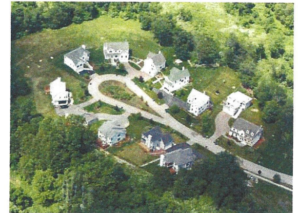
This neighborhood in Waterford, CT was constructed using multiple Low Impact Development techniques. Photo: Jordan Cove Urban Watershed Project, UCONN.
