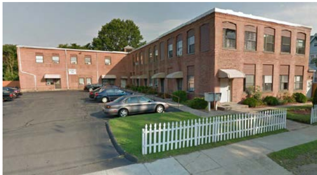
Existing apartment building at 180 North Cherry Street
