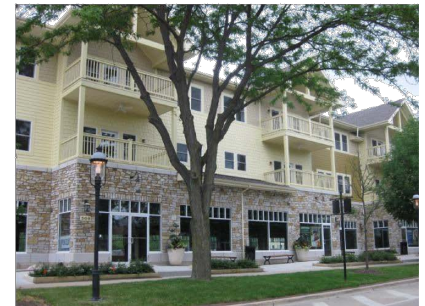
Mixed use building with ground level retail
