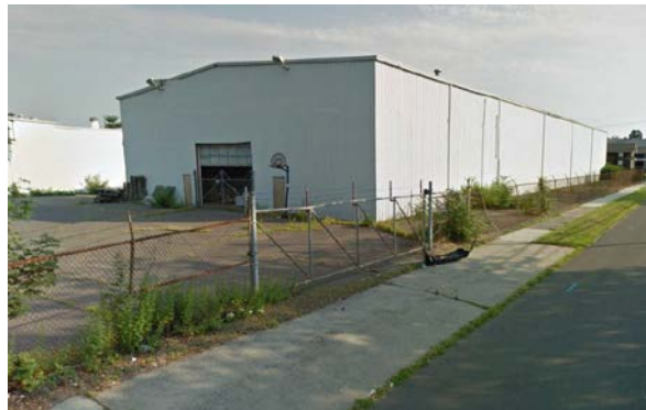
North Cherry Street: Blank walls line the street
