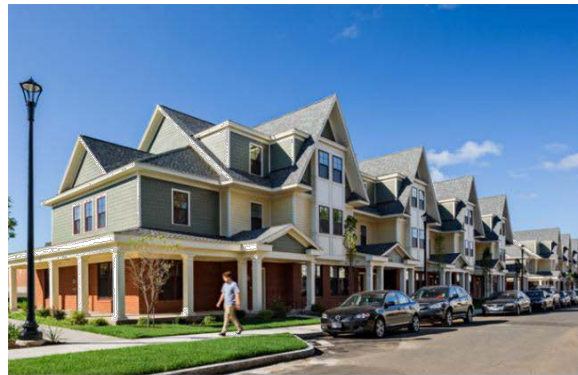
Apartment building oriented to the street
