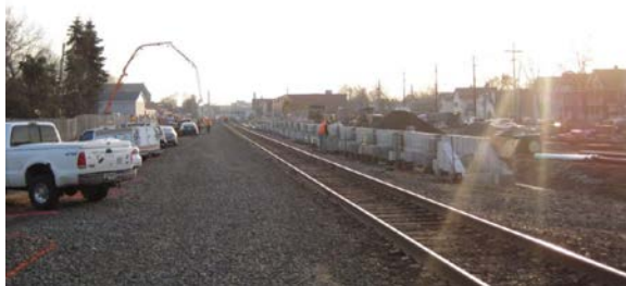
Platform construction on the west side of the rail corridor
