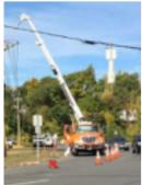
A typical day for linemen — when they aren't responding to emergency calls — can involve changing out poles that have been damaged or are beyond their useful life. Linemen inspect poles to see if there are any signs of rotted wood or water damage. Poles can also be damaged by falling trees or vehicle collisions.
